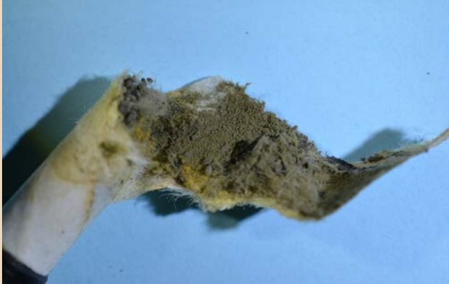
Figure 11. Plastic tubes are not recommended because they do not allow moisture to escape. Note water staining on outside of the cardboard liner and mold sporulating on the inside.
